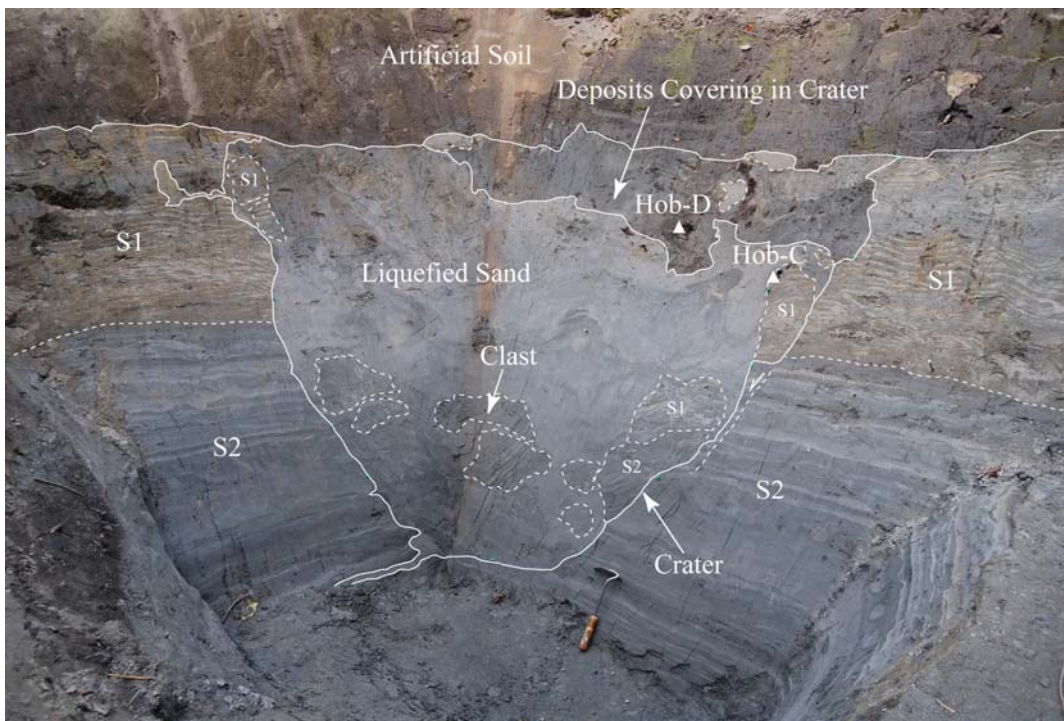
Figure 4-21 Crater confirmed at Hobigonj Village. S1: weathered alternation of silt and fine sand, S2: fresh alternation of silt and fine sand. Solid white line shows the outline of the crater. Broken white lines show clasts fallen down from the wall of crater. The clast in the center of the photo has inclined lamination, though the original structure of S1 and S2 is horizontal. The dark part on the top of the crater is deposits which covered the hollow after the eruption. Triangles represent the location of 14 C dating.
