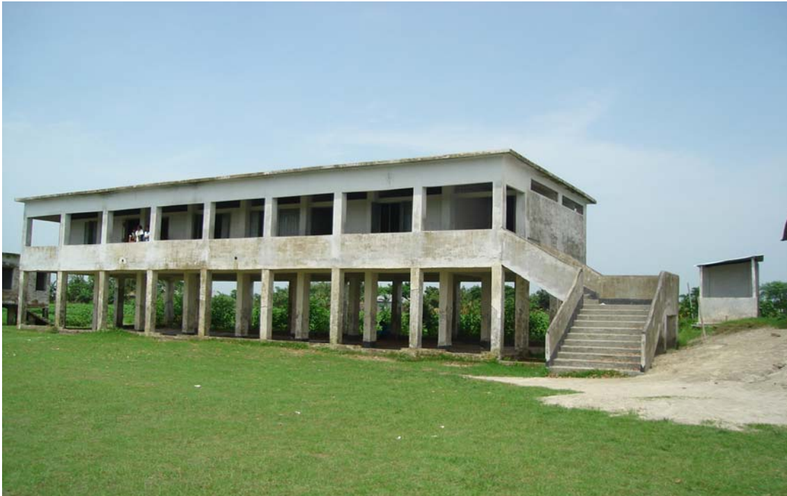
Figure-24: A Multi-purpose Cyclone Shelter, where the only Toilet is located outside
