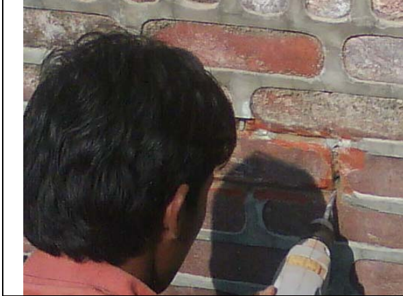
Drilling for removal of Masonry unit
