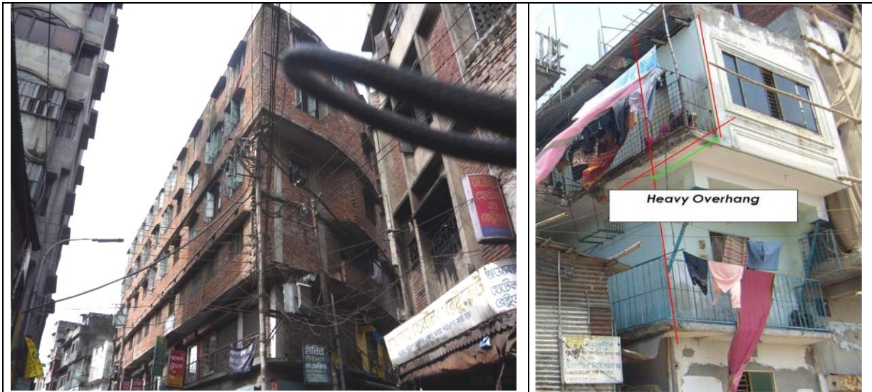
Figure 2-9 Typical Heavy Overhangs found in the old part of Dhaka City
