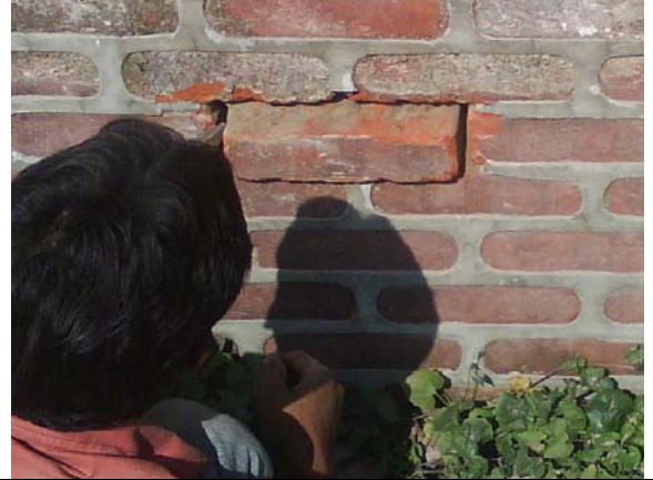
Removal Masonry unit
