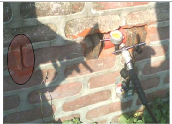
Giving pressure and measuring displacement
