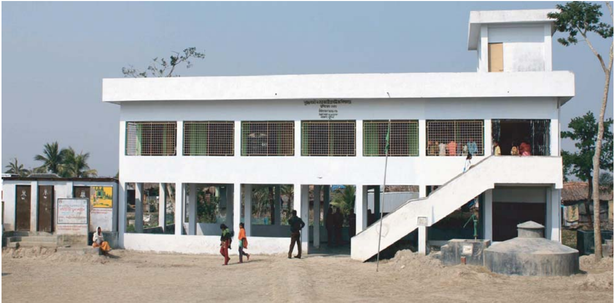
School cum cyclone shelter
