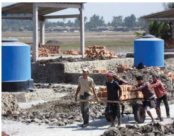
DRH Construction in progress
