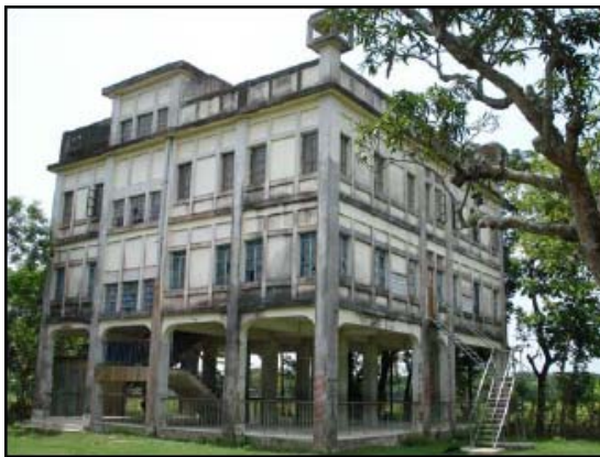
Figure 4.12: Type 11 cyclone shelter
