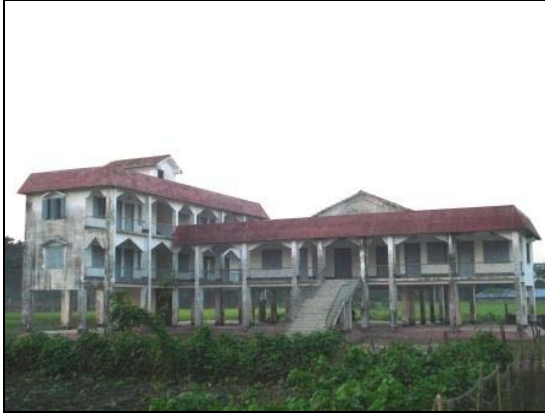
Figure 4.13: Type 12 cyclone shelter
