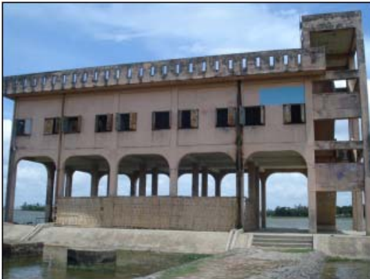
Figure 4.8: Type 7 cyclone shelter
