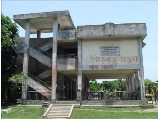
Figure 4.5: Type 4 cyclone shelter
