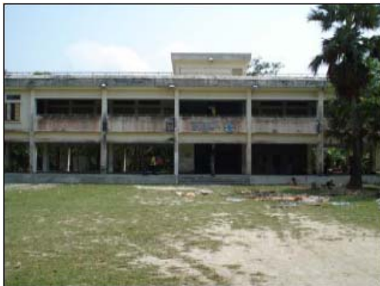
Figure 4.6: Type 5 cyclone shelter
