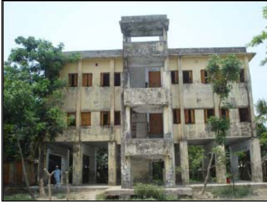
Figure 4.11: Type 10 cyclone shelter
