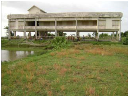
Figure 4.10: Type 9 cyclone shelter
