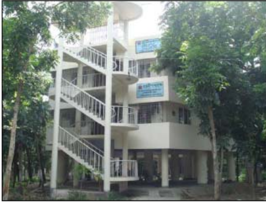
Figure 4.7: Type 6 cyclone shelter
