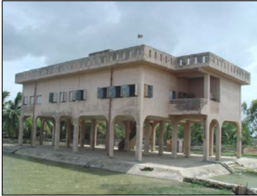
Figure 4.9: Type 8 cyclone shelter
