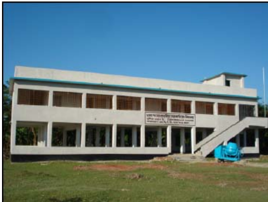
Figure 4.14: Type 13 cyclone shelter
