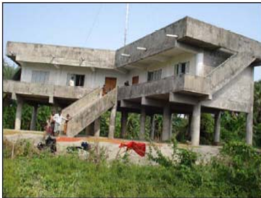
Figure 4.2: Type 1 cyclone shelter
