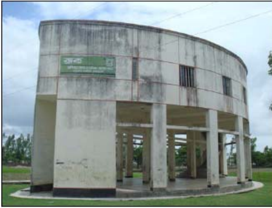
Figure 4.3: Type 2 cyclone shelter
