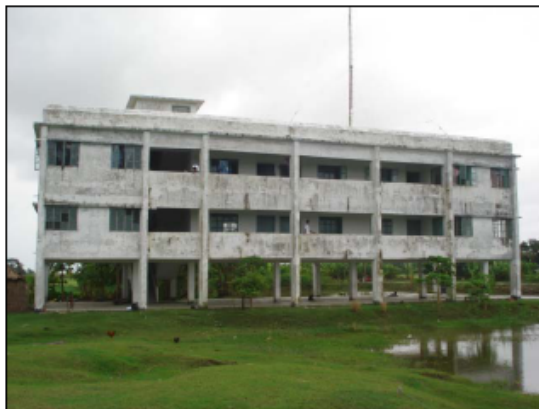
Figure 4.4: Type 3 cyclone shelter
