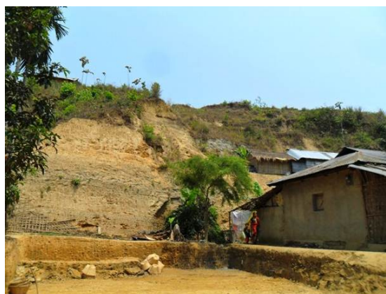
Vulnerable Houses at West Lar Para
