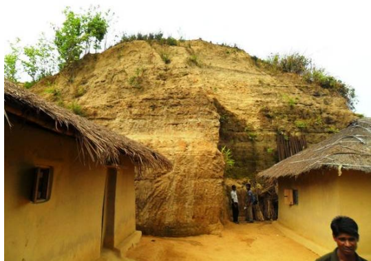
Vulnerable Houses at East Pahartoli
