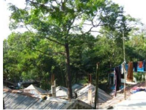
Houses vulnerable to Landslide-Mohajer para
