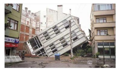
Foundation Weakening Due to Soil Liquefaction in Adapazari, Turkey
