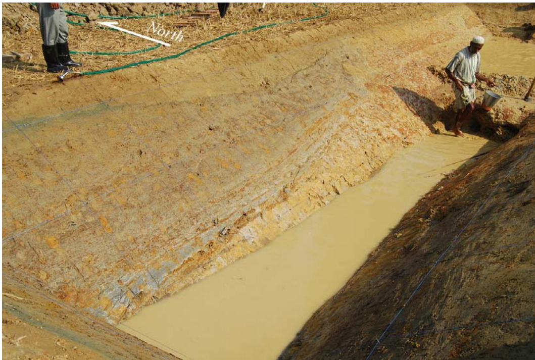
Figure 4-20 Photo of the North Wall of Feni-2 Trench taken from Southwest
