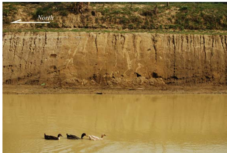
Figure 4-13 Sand Dikes at Awlatory Village
