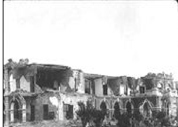
Court-Kachari Building Collapsed at Mymensing after 1897 Earthquake
