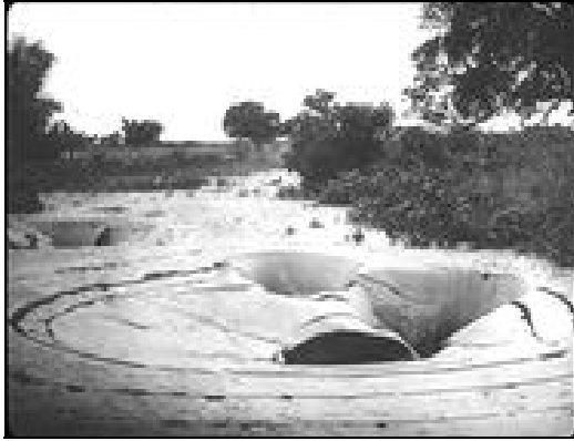
Sand vent at Rowmari, 1897 Earthquake
