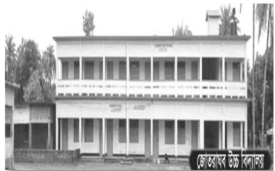
Figure1.8: School cum shelter
