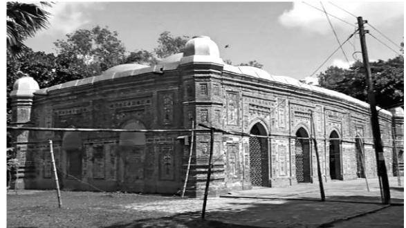
Figure1.9: Bagha shashi mosque
