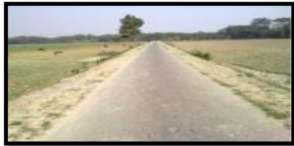
Fig 1.2: Basbaria via Dashomina Road
