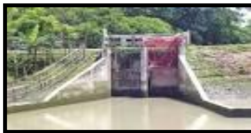
Fig 1.1: Sluice Gate of Dashomina
