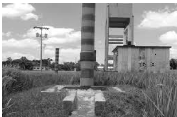
Figure1.5:Deep tubewell under borendro irrigation project
