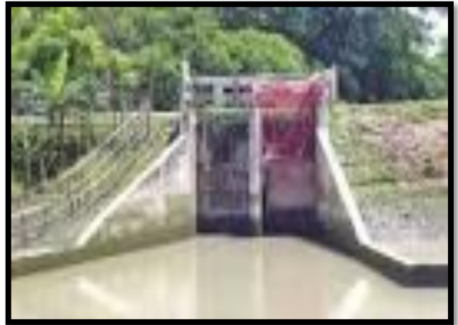
Photo1.2: Sluice Gate Golachipa
