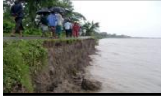
Photo 2.5: River erosion are Tentulia River.
