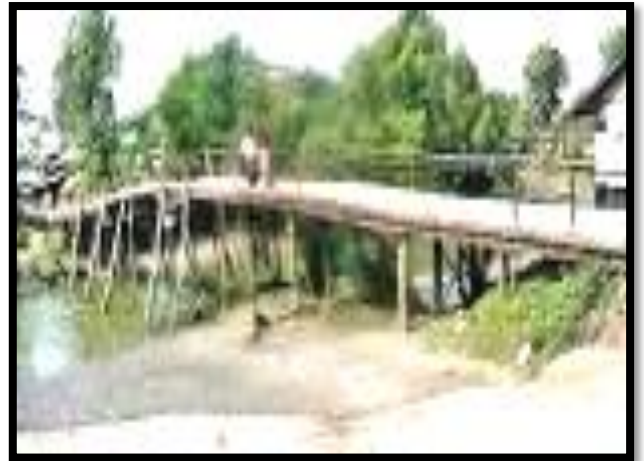
Photo 1.3: Bridge and Culvert Golachipa
