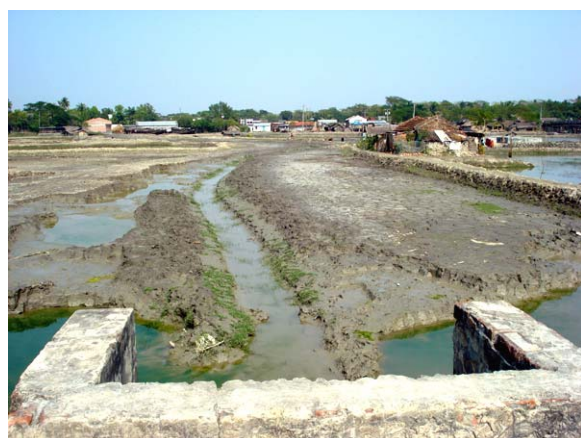
Figure B.8.6.a: Siltation on Kobadak river leading to closure of sluice gate
