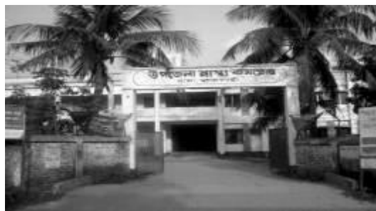
Figure 1.11: Health Complex in Bagha
