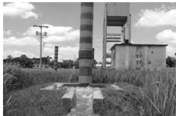
Figure1.4: Deep tubewell under borendro irrigation project
