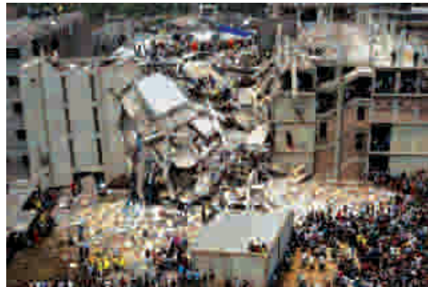
Rana plaza after collapse, Photo Credit: http://img.wikinut.com/img/3yx0v86i3it_mqyd/jpeg/0/Rana-Plaza-Collapse.jpeg
