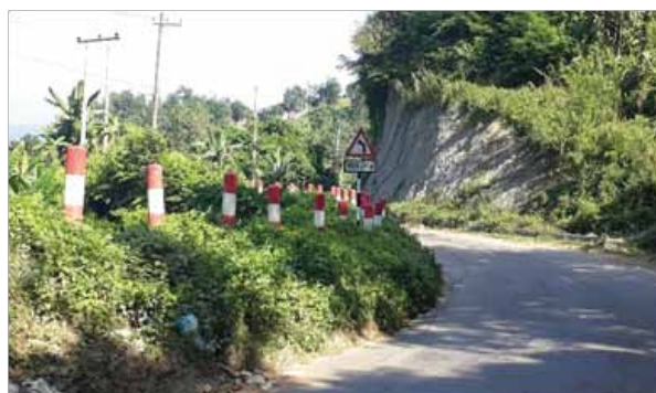
Photo 2: Unstable uphill slope close to roadway
