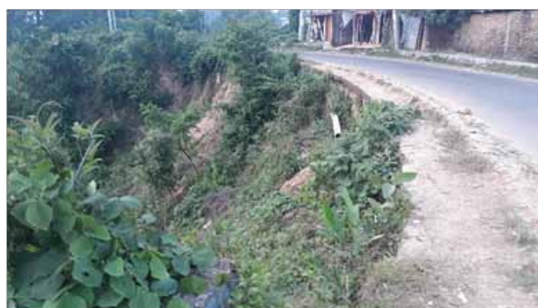
Photo 5.3: Damaged downhill slopes of roadway
